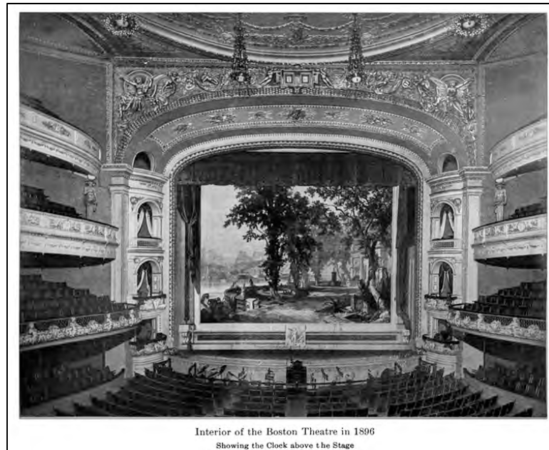
Fig. 3.9 Boston Theatre in 1896 showing the arrangement of seats and separation of tiers. The seats are replacements installed in 1896. The wire fronted first tier balcony can clearly be seen, but seats in the top tier gallery are almost invisible. Private boxes are limited to six boxes on the sides of the proscenium, seated with moveable parlor chairs. (Tompkins, The History of the Boston Theatre 1854-1901 , 1908, 431)
